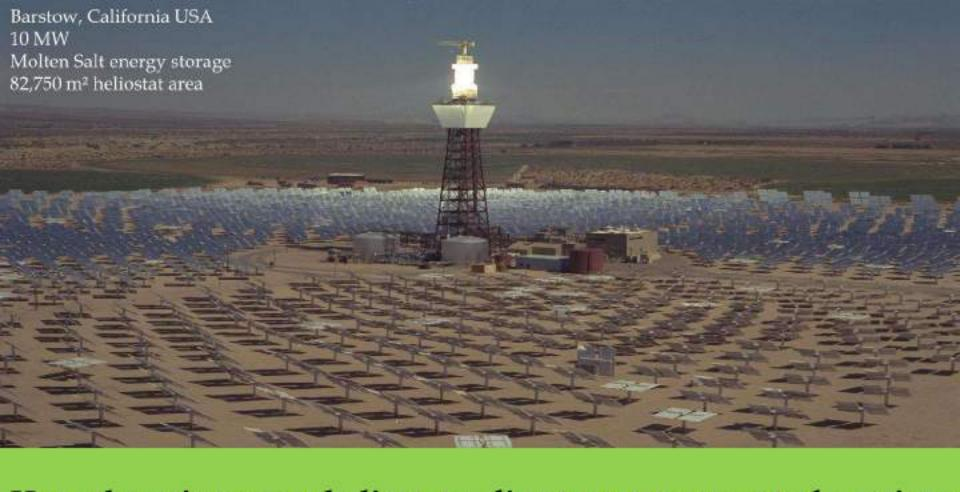
Here the mirrors, or heliostats, direct rays to a central receiver where a molten salt absorbs heat. This plant produced 10 MW until its decommissioning in 1999. This is obviously a large scale, centralized power plant connected to a massive electrical grid, which contrasts with PV panels which can be placed remotely.
